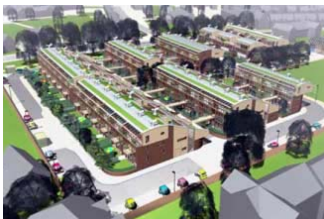
03 - ZEDfactory team propose an additional 1,550m² net workspace on the same 0.64 ha plot. Density is 203 workspaces / ha @ 12m² / workspace, with car pool shared with housing
